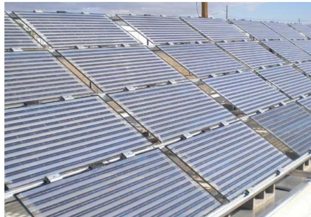
**Figure 1. The holographic concentrator PV system made by Prism Solar Technologies, Inc. The modules are 20 x 32 inches, and feature holographic diffraction gratings embedded within each module between strips of PV cells.**
